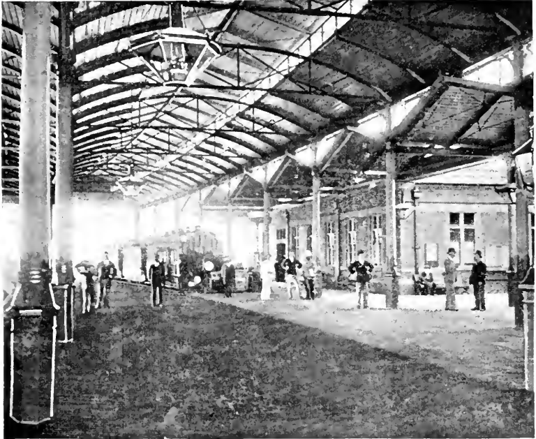
INTERIOR OF RAILWAY STATION, MARITZBURG.
